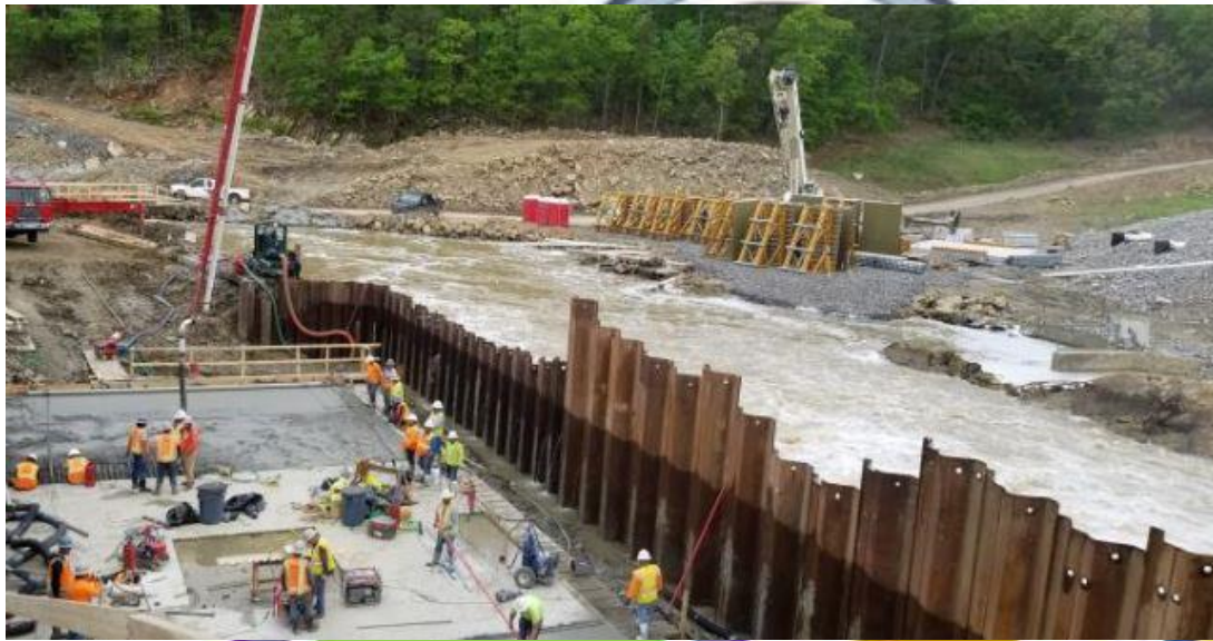
Atoka Dam Rehab
